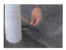
**Step 1**- Cut a hole in the PondGard panel that is approximately 75% of the outside diameter of the pipe protruding from the substrate.
