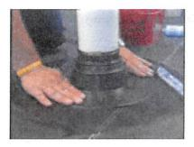
**Step 10**- Smooth the pipe boot flange onto the PondGard panel.
