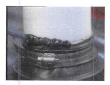
**Step 13**- Apply a continuous bead of Lap Sealant HS or All Purpose Sealant over the top edges and the edges at the base of the boot.
