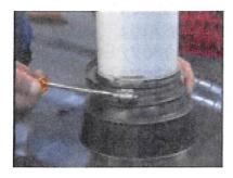
**Step 12**- Attach and tighten the stainless steel clamp to the pipe boot rib that grips the pipe.
