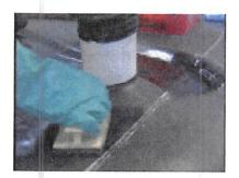
**Step 5**- Using a scrubber pad and holder; apply QuickPrime™ Plus Primer to a 14.0" (35.56 cm) diameter area around the pipe. Make sure to extend primer past the adhered pipe boot flange area.
